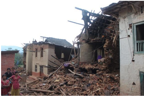
90% houses were collapsed in Baluwa Village
